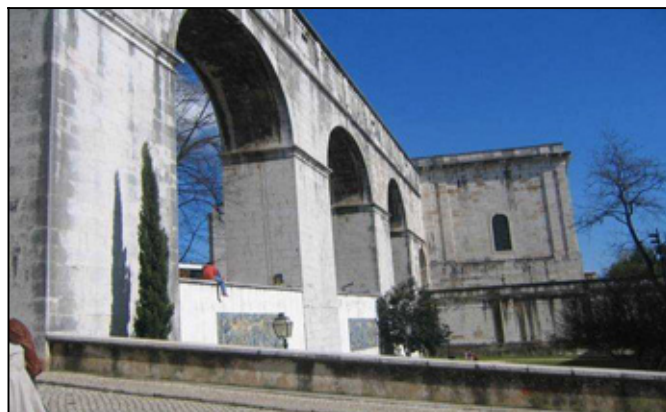
The Lisbon end of the aqueduct.
