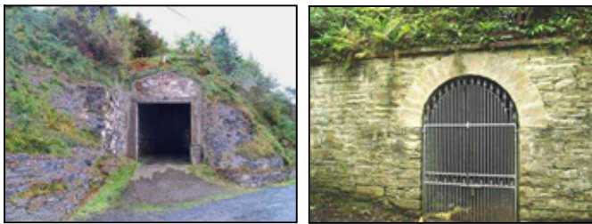
Left - North end of tunnel. The ornate portal was removed during road widening. Right - Exit from side tunnel to stables.
