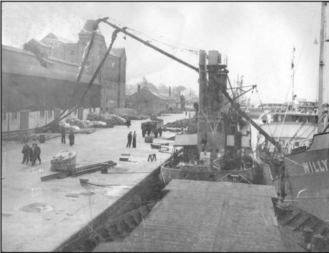
This photograph by George Spillane shows the Garryowen doing the reverse of what it normally did – sucking grain out of Rank's silo at Limerick Docks and blowing it into the coaster at right.
