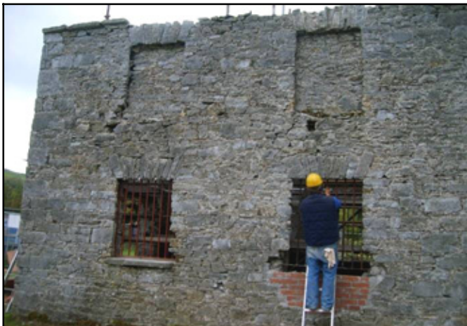
Consolidation work in progress at Ballincollig, March 2010.
