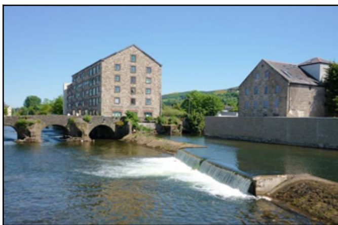
The Old Bridge across the Suir to Suir Island. The weir in the foreground supplied a flour mill at centre, now rebuilt as apartments.
