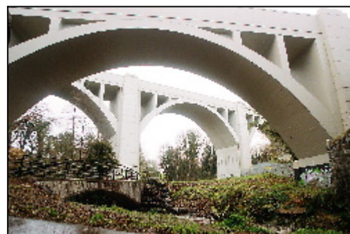
Bleach Green Viaducts
