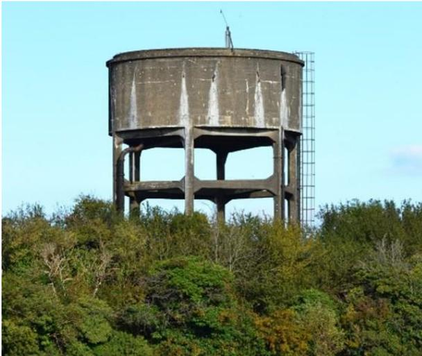
15in. square legs each have a 7ft sq. pad foundation, all six pads being connected by a "wheel" of ground beams. At 10ft vertical intervals, the 30ft long legs are braced by a ring beam 12in. by 9in. section. Inside the legs are cross-braced in a triangle, a different set of legs being so braced at each level. The tower was cement gunited (sprayed) in recent times to halt corrosion of the reinforcement.
