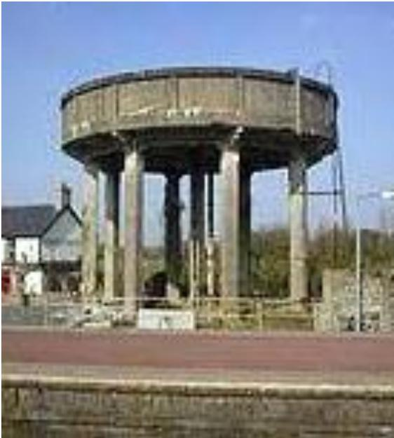
A large shallow free-standing circular tower in concrete, constructed in 1950 and probably a replacement for an earlier tower, is located at Ballybrophy station in county Laois.
