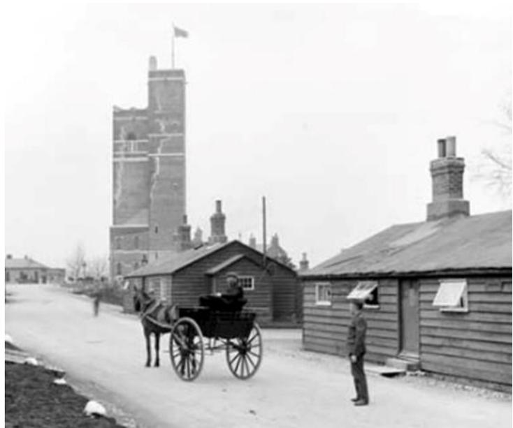
***On the left, the reinforced concrete water tower at St Joseph's hospital in Limerick and on the right the military camp on the flat plain of the Curragh in county Kildare, an ideal candidate for a water tower as the photograph indicates. The tower at the Curragh was built in brick between 1900 and 1908. The camp fire-brigade is based in the tower, making it one of the earliest purpose-built stations in the country.***
