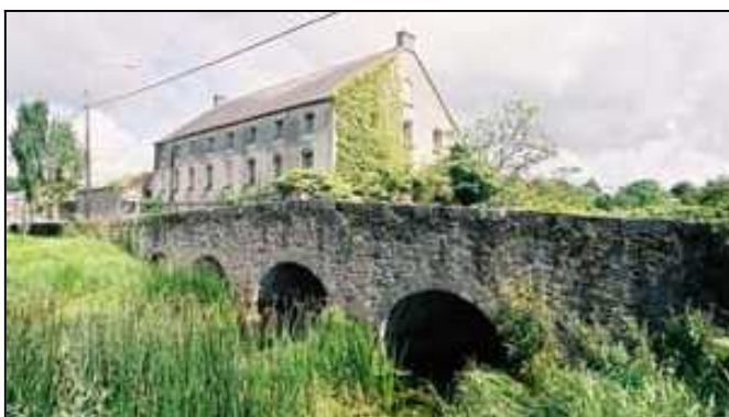
Mid 18 th century bridge over River Brosna at Clara.
