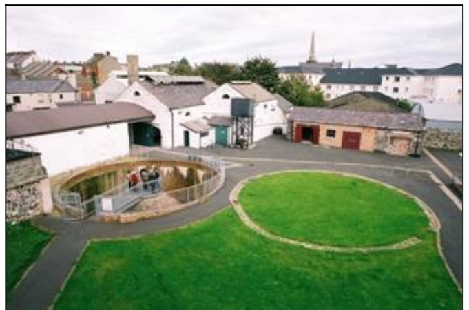
Carrickfergus Gasworks as seen from the gasholder. The buildings at top left house 36 horizontal retorts in which the gas was made.
